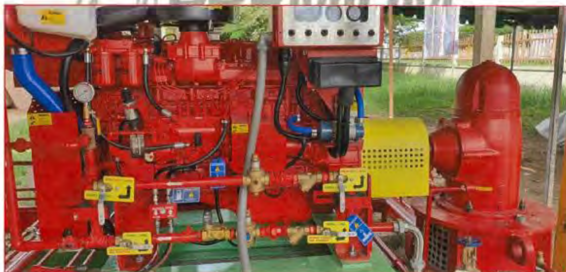
Diesel Engine Fire Pump
